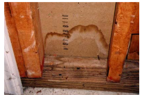
The obvious evidence of water damage to this basement wall is a sure indication that a mold problem is likely to develop if the situation isn't corrected.
